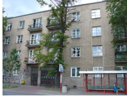
The apartment block at no 6 Boboli St in Mokotow. Picture taken in 2006
