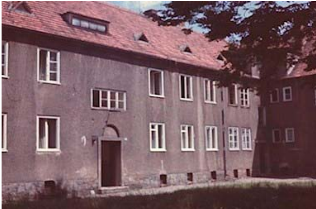
The house where we lived. The open door led to four apartments. Ours was upstairs, the three windows on the right.
